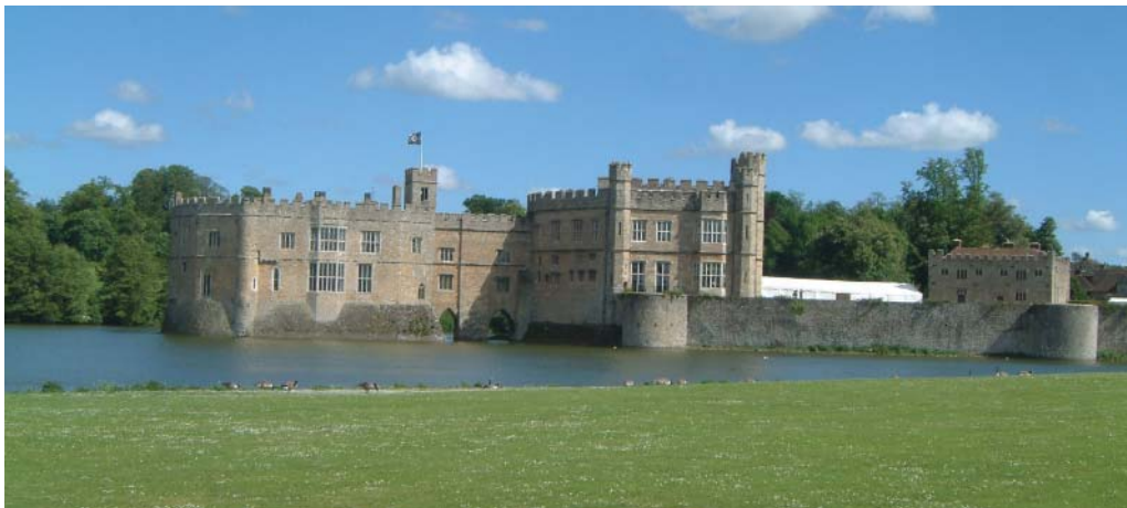
FIG. 5. Leeds castle, Kent. The gloriette , on its own separate island, occupies the left side of the photo. The distance between the water surface at the base of the gloriette and the windows of its ground floor indicates that the ground floor is at least 2 m above the lake level
