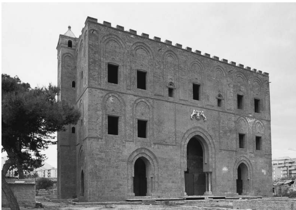
FIG. 3. La Zisa of Palermo: east façade. The tower abutting the south façade is visible at the left end of the pavilion. On the east façade, the two levels of windows above the ground floor demonstrate that the structure has three levels. The window openings, which are modern, differ from the originals
